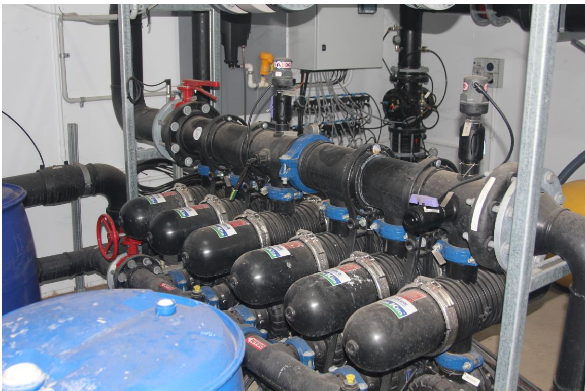
Figure 17: A bank of disc filters in a complex irrigation system (Photo: Pinion Advisory)
