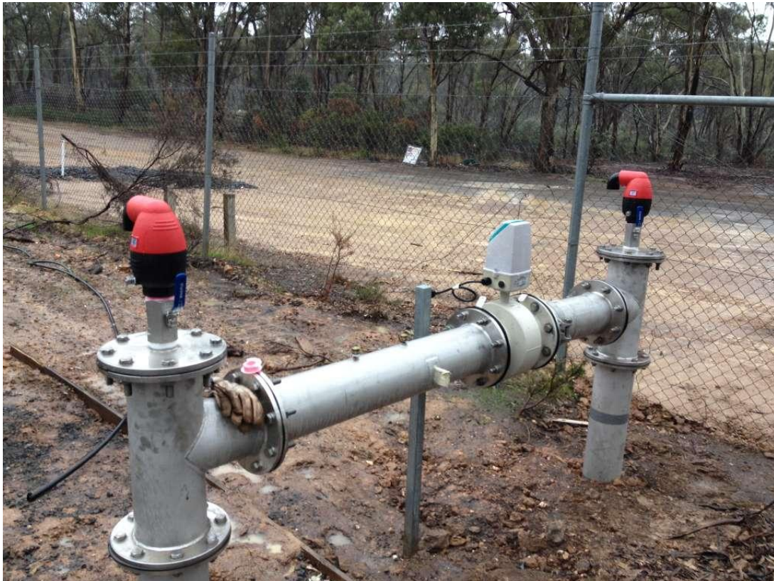
Figure 20: Air release valves (Photo: (Bermad Water Technologies, 2018))
