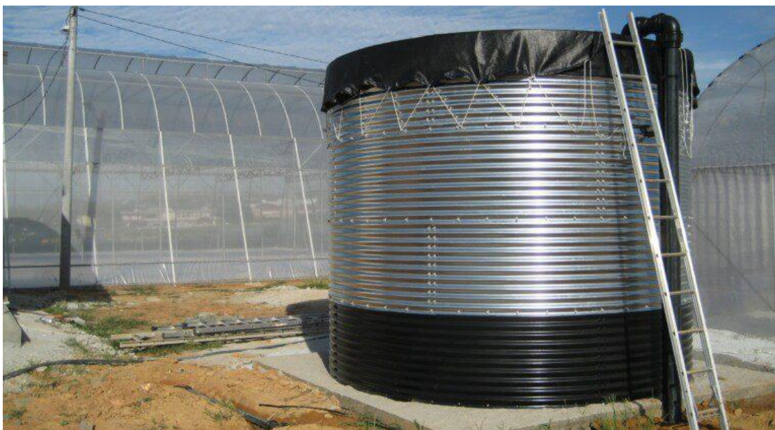
Figure 15: Tanks are used as backup water supply in substrate based production (Photo: (NPI Water Storage, 2025))
