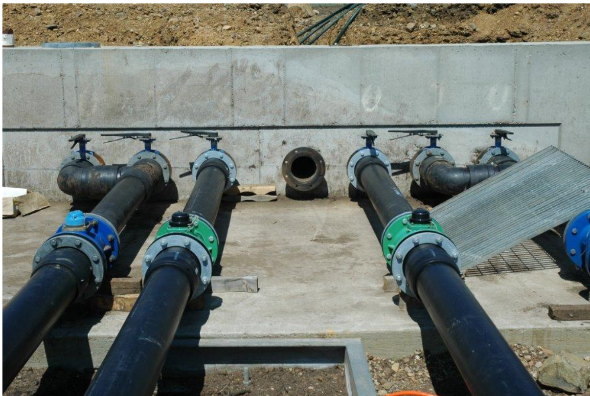
Figure 20: These pipes are made of polyethylene (Photo: Pinion Advisory)
