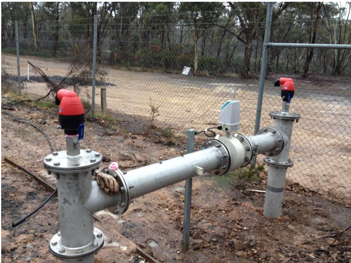
Figure 22: Air release valves (Photo: (Bermad Water Technologies, 2018))
