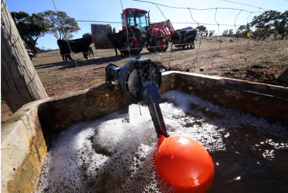
Figure 27: Float valve (Photo: (Land and Water Technology, 2025))
