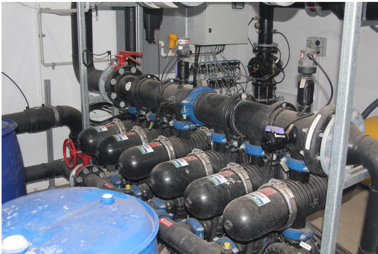
Figure 19: A bank of disc filters in a complex irrigation system (Photo: Pinion Advisory)
