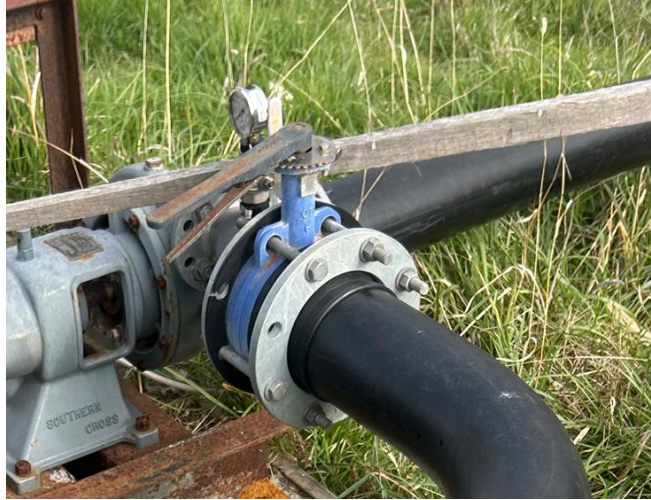
Figure 25: Butterfly valve (Photo: Pinion Advisory)
